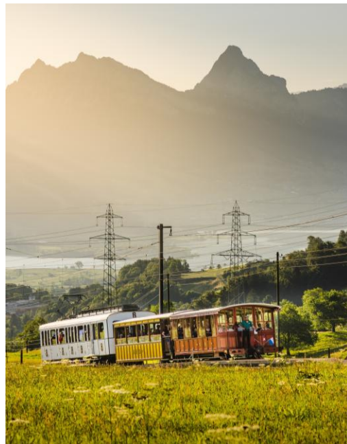
Train No. 6 (1911), oldest electric train worldwide, with wagon No.35 (1899) and No. 5 (1871!!)
